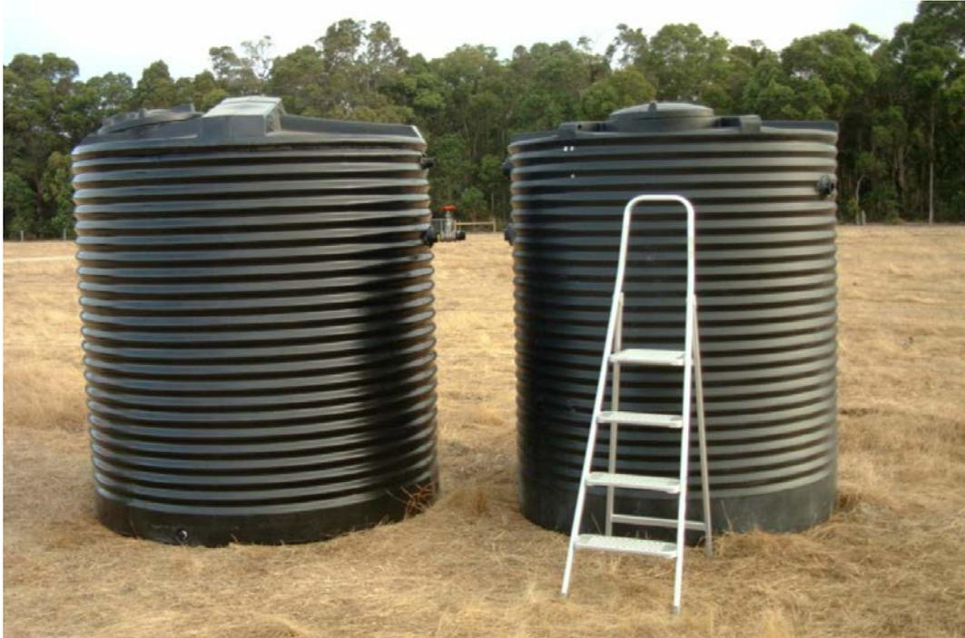
Figure 2: 4500 L filter tank (left) and 3500 L reservoir tank (right)
