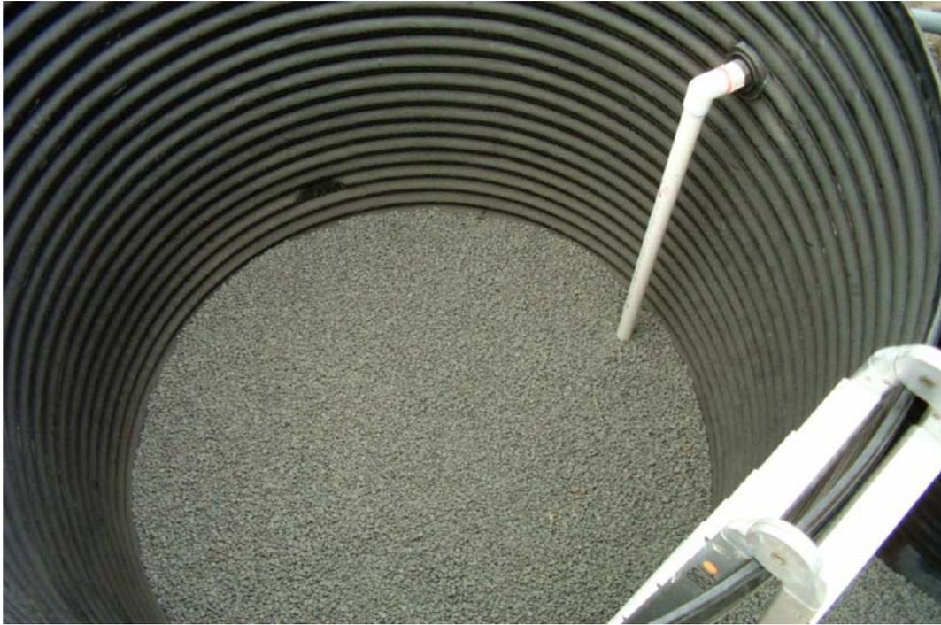
**Figure 5: The bottom layer of gravel is in place. The pipe assembly is embedded in it. On the right side is the rising pipe that transports the collected water up and over into the reservoir tank.**
