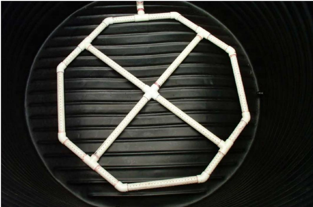
Figure 4: The collecting pipe assembly in place at the bottom of the filter tank, before it is embedded in a layer of gravel (see text for details)
