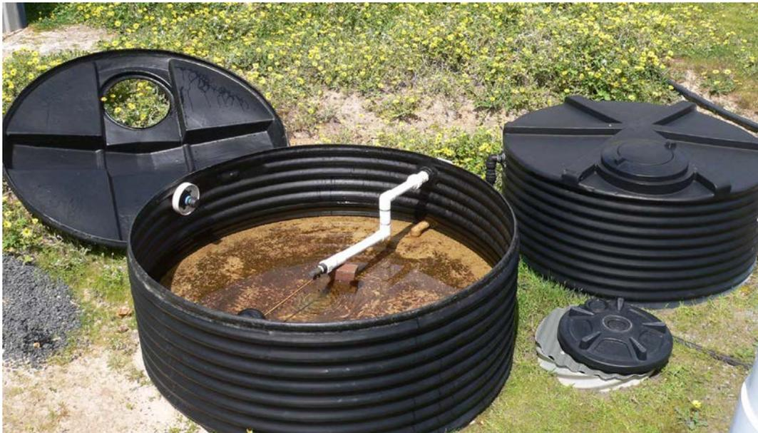
Figure 7: The reservoir tank (right) is equipped with a 40 cm man-hole, which only allows limited (but sufficient) access to the inside of the tank. In contrast, the entire top of the filter tank (left) needs to be removable to build the filter, and for maintenance purpose. The inlet of fresh, unfiltered water to the filter tank is controlled by a simple float valve (see text for explanation)
