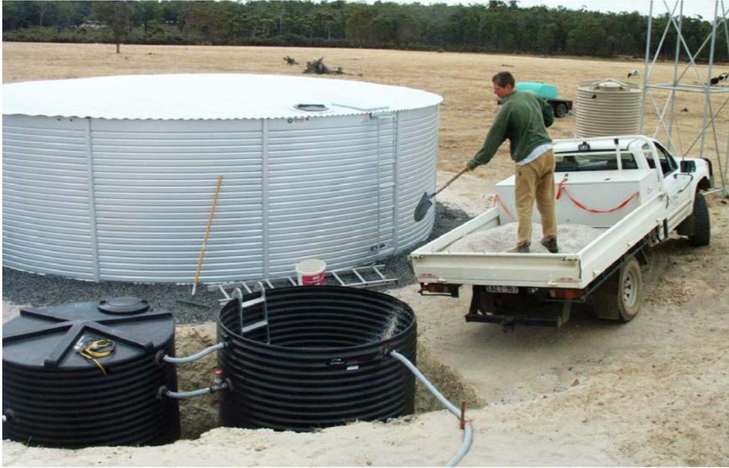
Figure 6: Filling the filter tank with lime sand.
